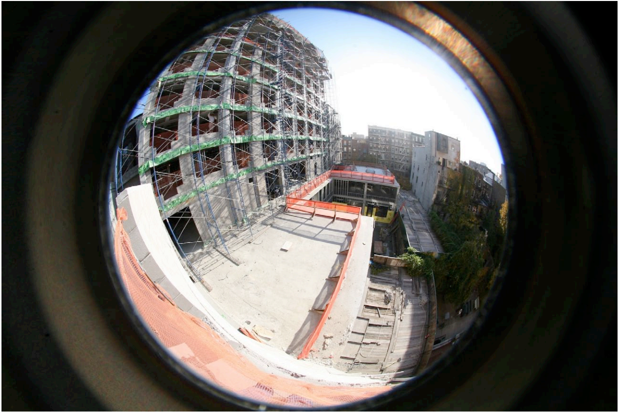
View of the 3rd Floor Girls Club Green Rooftops
